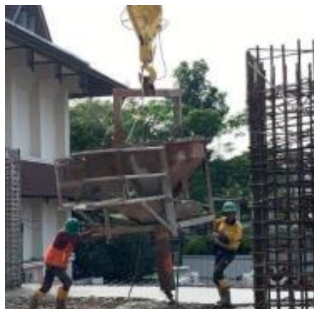
Gambar 3.37 Concrete Bucket Cor
