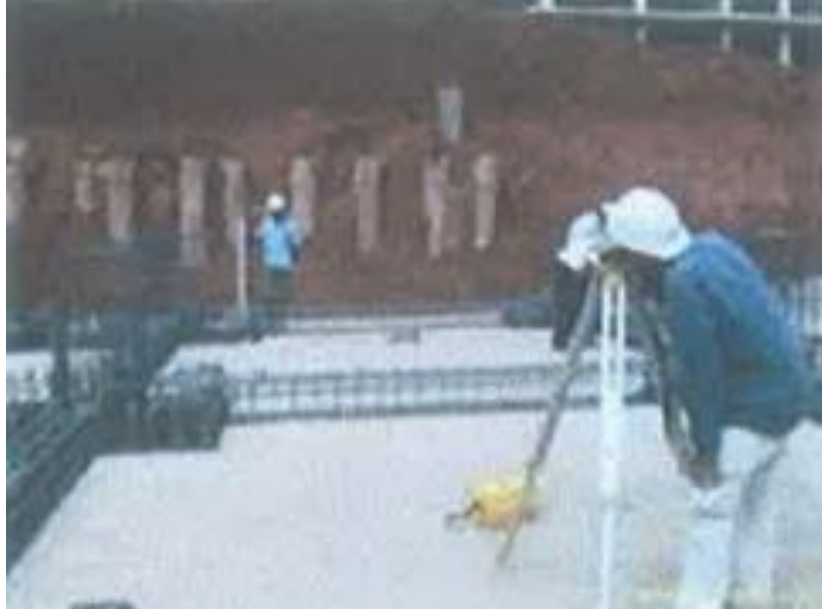
Gambar 3.66 Penentuan As Kolom
